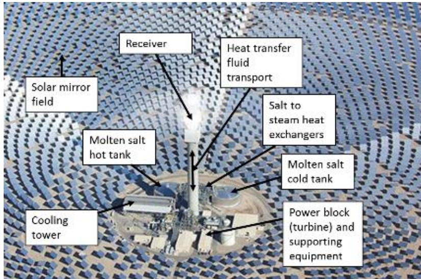
Figure 2: Subsystems in a molten salt tower plant.
