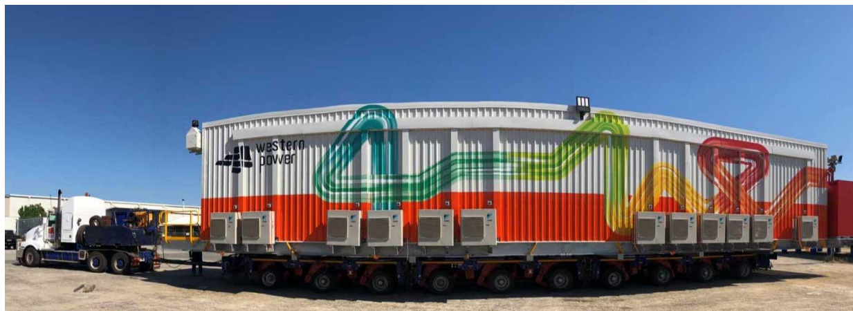
Figure 49 Kalbarri battery being transported from Perth 126
