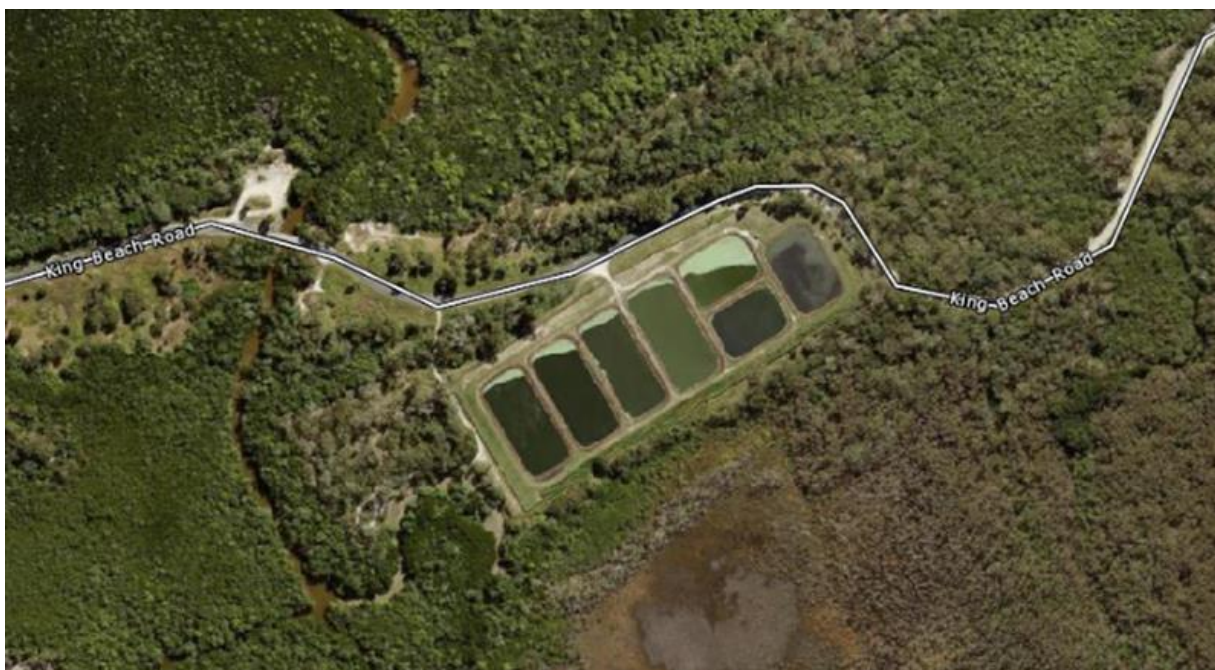
Figure 38 Yarrabah Sewerage Treatment Ponds
