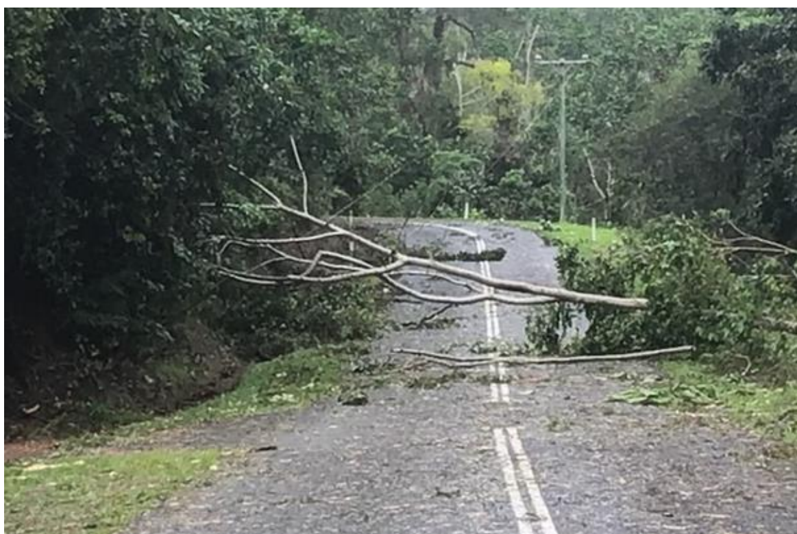
Figure 18 Typical powerline damage indicative of cyclonic activity
