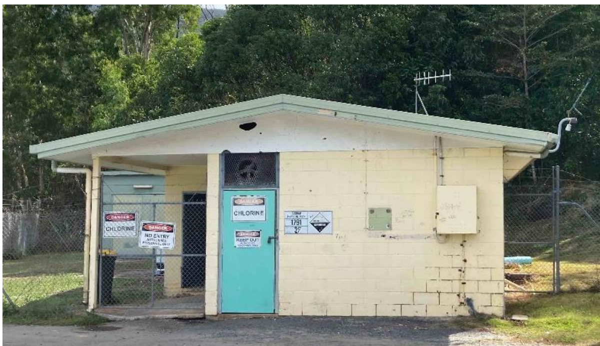
Figure 37 Yarrabah Water Treatment Station
