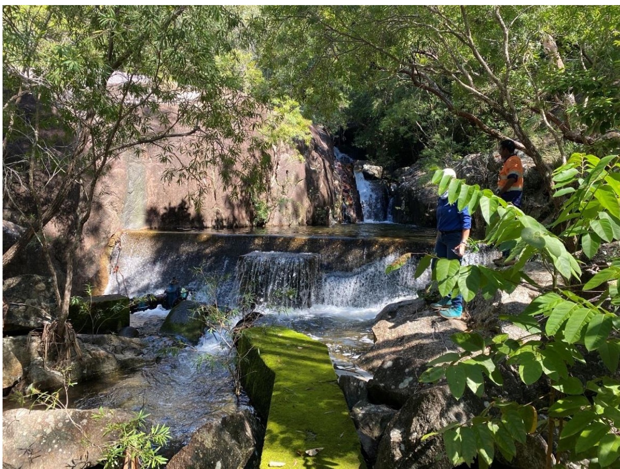
Figure 35 Old water intake structure at Reeves Creek - no longer used
